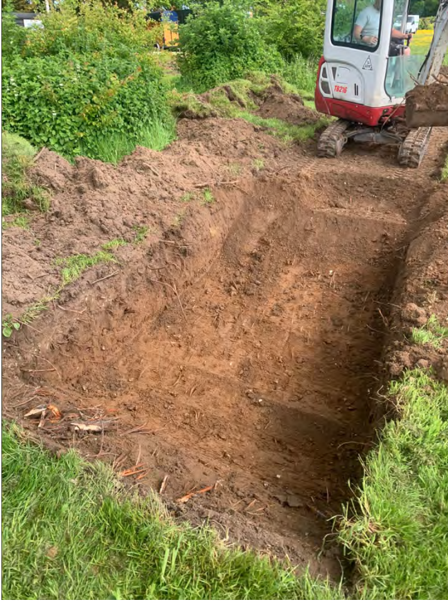
Plate 2, North facing working shot - machine excavation of Trench 2
